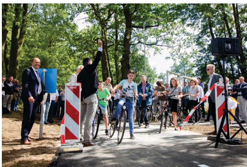
Figure 25. A cycle track with lignin asphalt was opened at the Wageningen University Campus in 2017 (photograph: Marte Hofsteenge).
