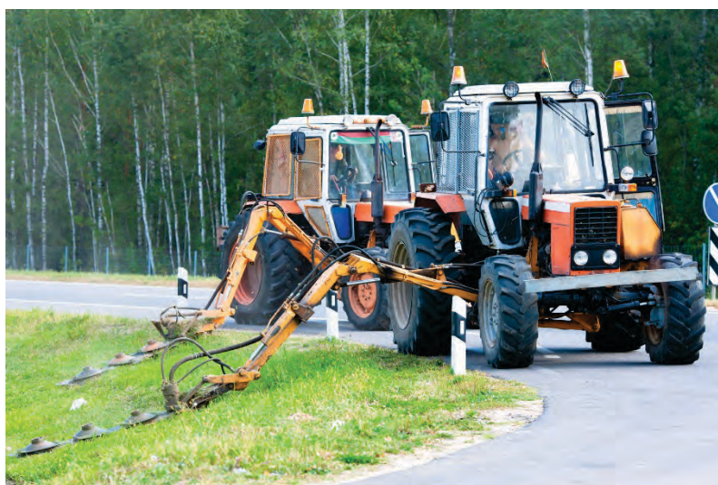
Figure 20. Verge grass can be used in a pyrolysis process.
