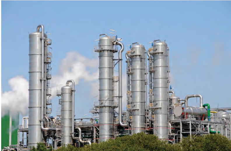
Figure 16. Bioethanol plant located at the Maasvlakte, Port of Rotterdam.
